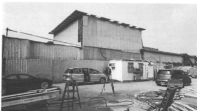
Photo No. 2 Viewing to the south side, along the boundary is the metal fence. Beyond is sheltered temporary warehouses with ground level at +20.50mPD to +20.01 mPD.
