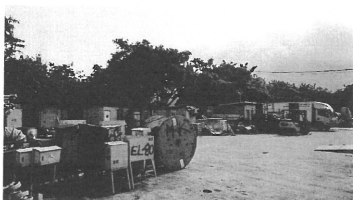
Photo No. 6 To the north of the proposed site area. It will be covered with metal shelters for warehouse.
