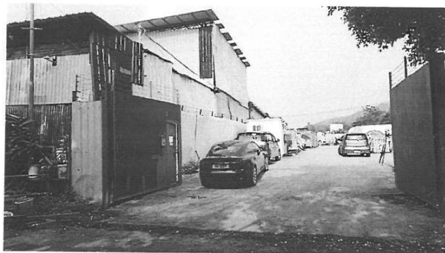
Photo No. 1 Viewing to the front side the proposed site entrance. It is an existing 300mm U-channel crossing. The site is a paved area around +20.5 mPD. Other four sides outside the site boundary are also in a flat area, similar ground level in comparing to the proposed site.
